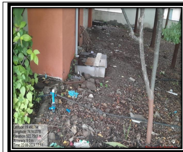
Rain Water Harvesting
